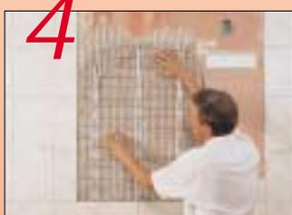
Press the mirror heating mat into the tile adhesive – make sure it is even and fixed. Then cover the mat with tile adhesive – make sure the surface is smooth.
