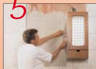
Put the connection tail of the mat into the flex pipe and push it up to the connection box.
